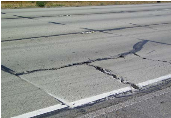
Figure 320-5: Replace slab and base – 3 rd stage cracking \geq \frac{3}{4} " wide, settlement \geq \frac{1}{4} ", spalling
