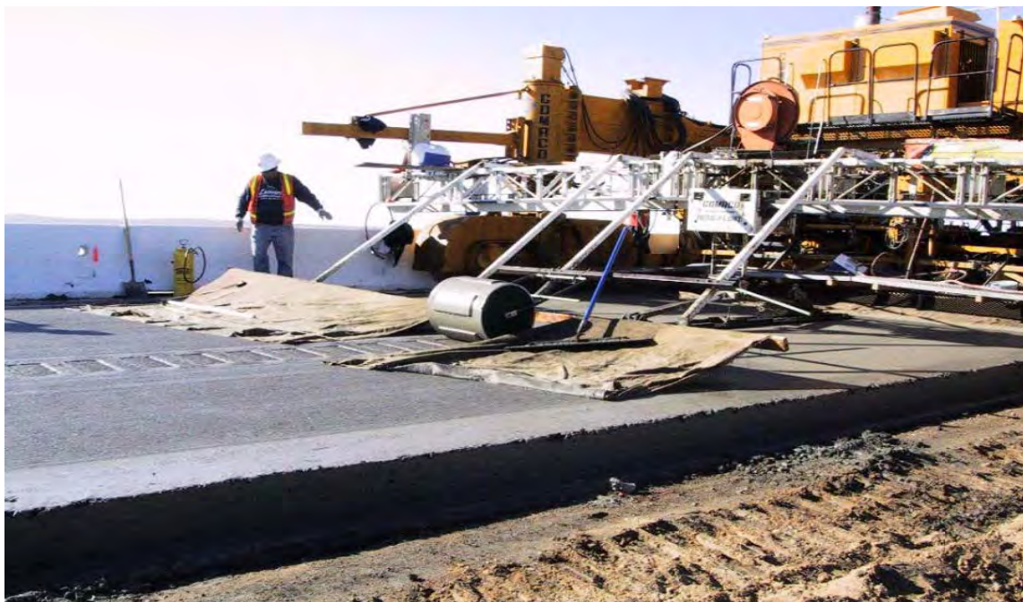
Figure 420-2: Unbonded concrete overlay construction
