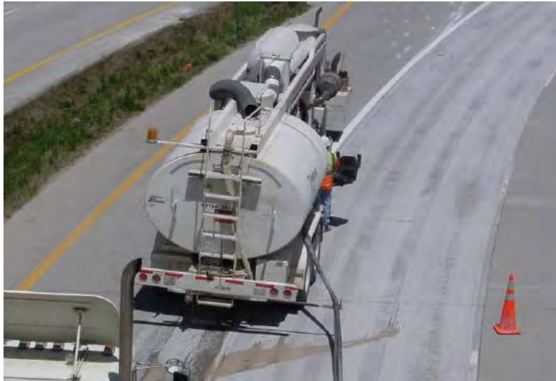
Figure 340–5: Grinding residue collection
