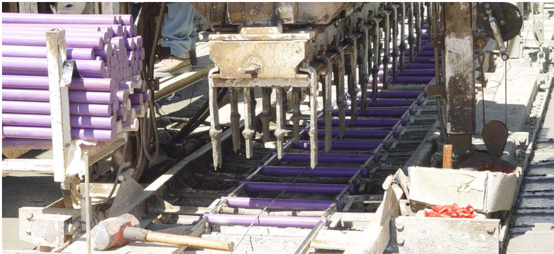
Figure 210–5: Dowel Bars
