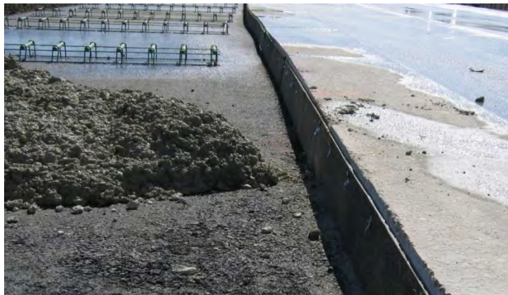
Figure 400-2: Isolation joint
