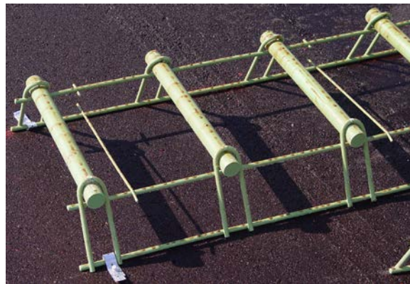
Figure 120-5: Dowel bars
