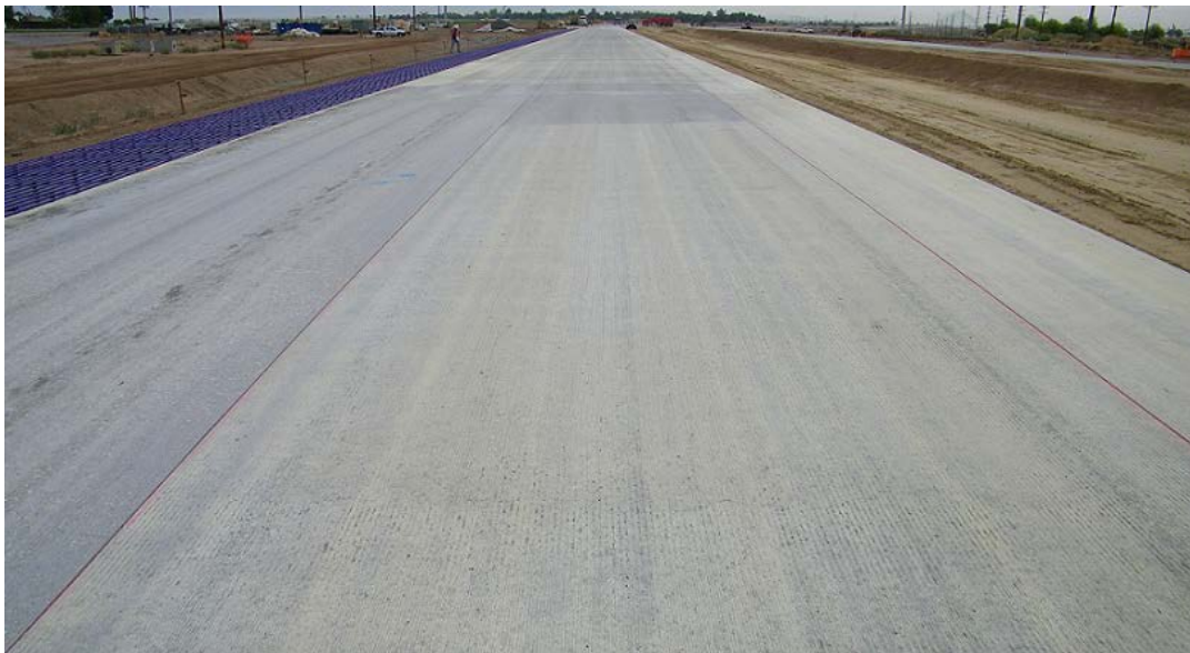
Figure 200–6: Longitudinal contraction joints
