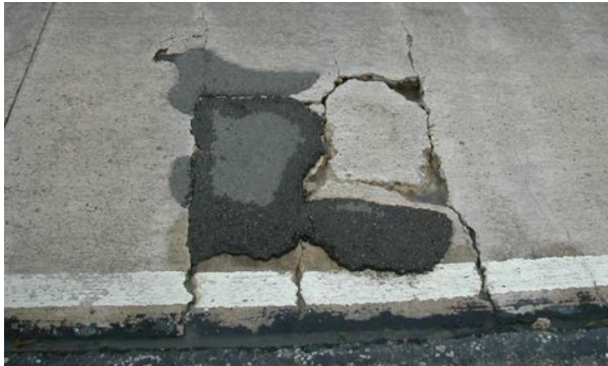
Figure 200–10: Typical edge punchout
