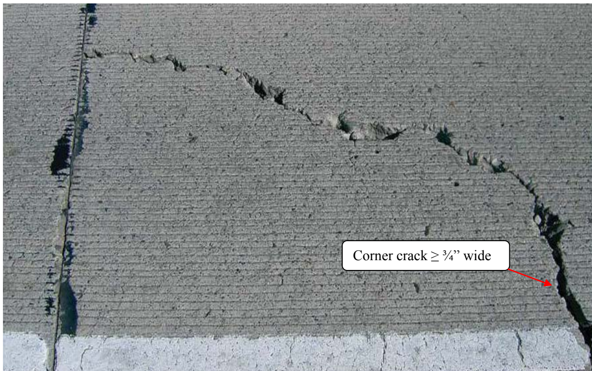
Figure 320-2: Replace slab – severe corner crack ≥ ¾” wide
