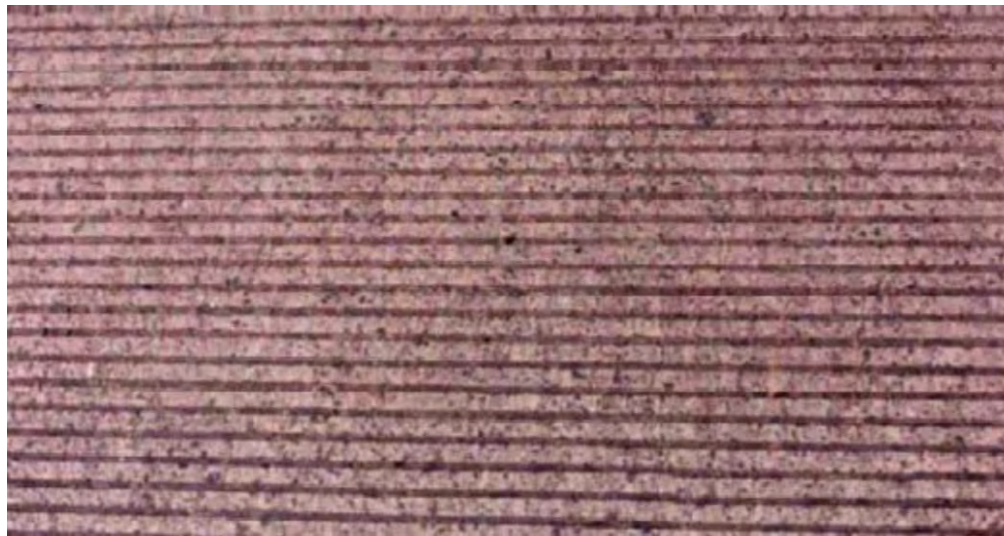
Figure 340-4: Grooved pavement surface
