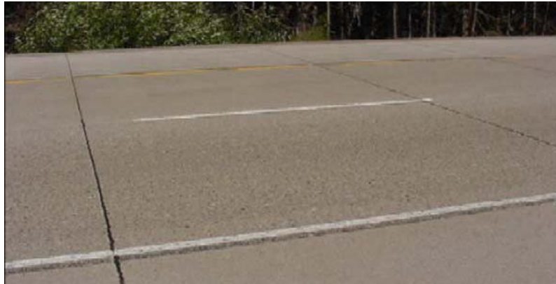
Figure 210–2: Transverse and longitudinal joints
