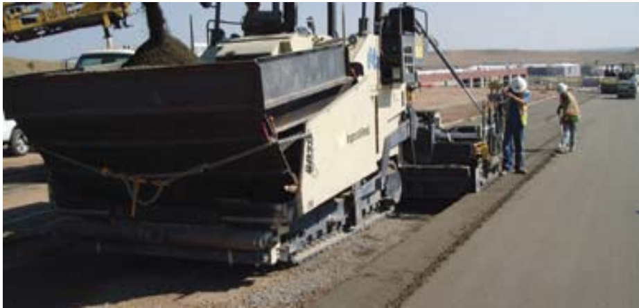
Figure 120–3: RCC pavement construction (NCPTC, 2010)
