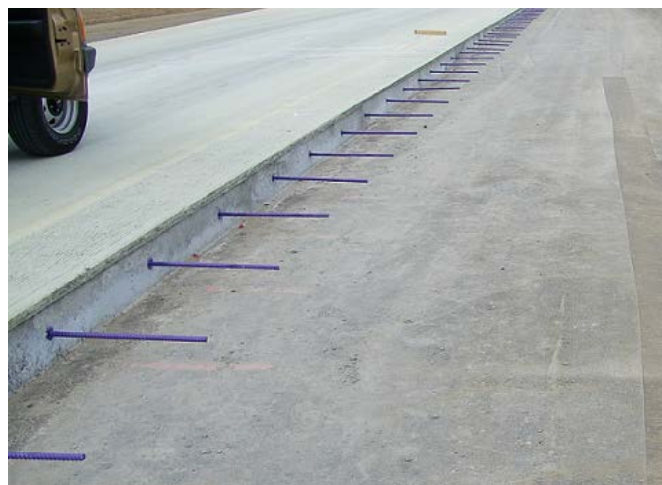
Figure 200-5: Longitudinal construction joint
