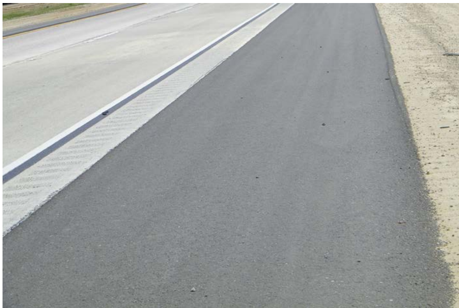
Figure 200–11: Widened CRCP lane with HMA shoulder
