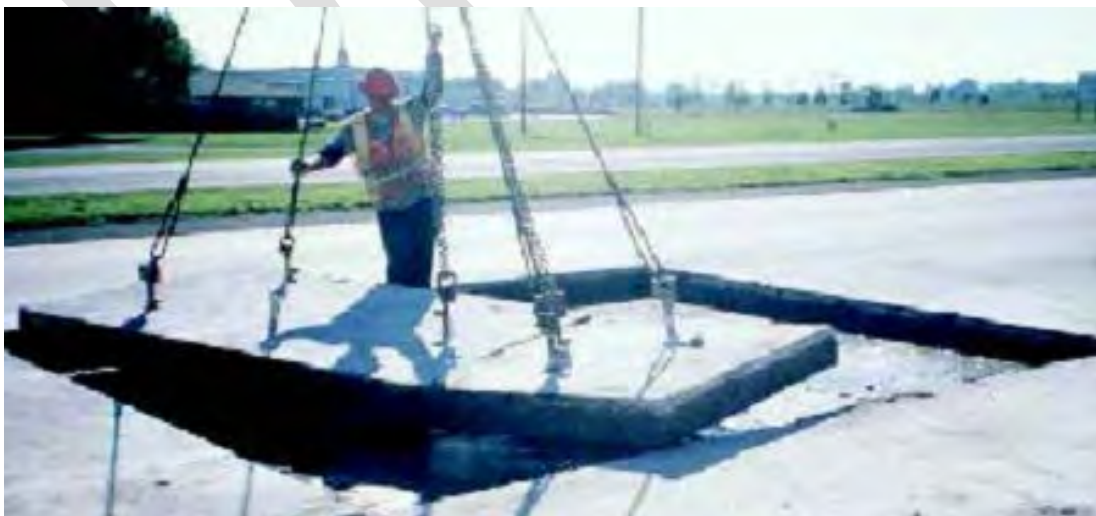
Figure 380-3: Concrete removal using lift-out method
