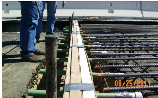
Figure 200–7: Expansion joint
