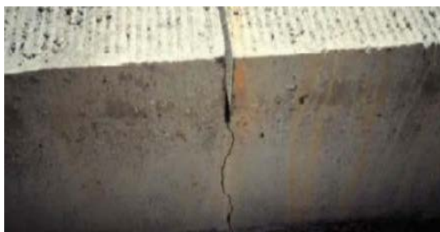
Figure 120-6: Aggregate interlock at a transverse joint
