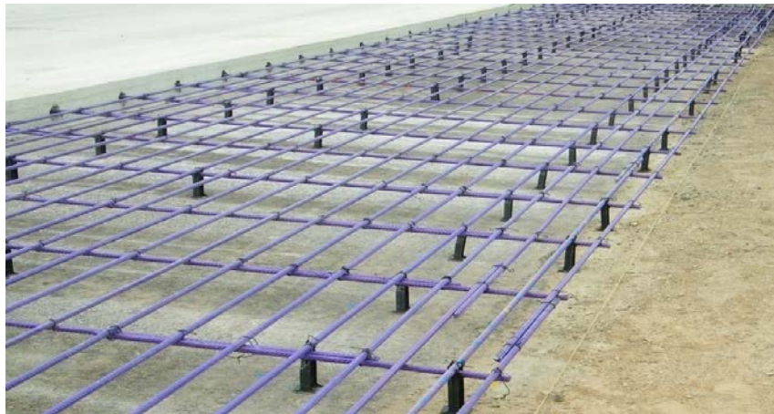
Figure 200–1: Epoxy coated CRCP reinforcement
