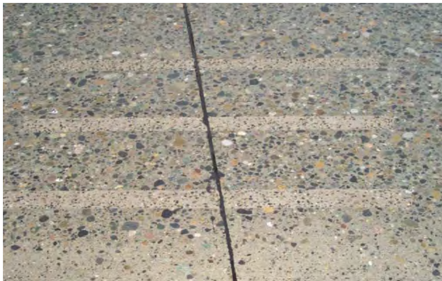
Figure 330-1: Completed dowel bar retrofit (single wheel path shown)
