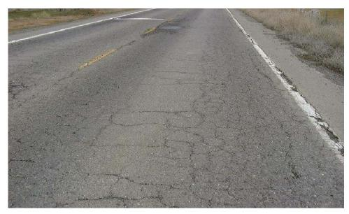
Figure 4. Structurally Inadequate Pavement (severe alligator cracking and rutting distress)
