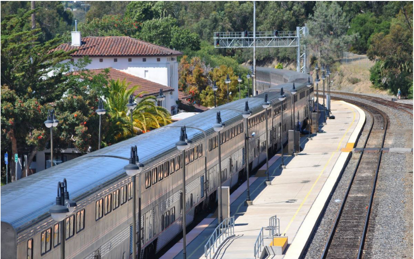
San Luis Obispo Station (Source: wikimedia commons, https://upload.wikimedia.org/wikipedia/commons/6/6a/San_Luis_Obispo_Amtrak_Station_Ca._-panoramio.jpg )
