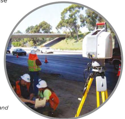
*Caltrans District 11 crew surveys the Highway 805 and 905 interchange using a ScanStation 2 laser scanner during training.*
