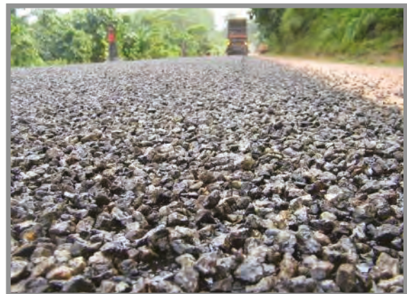
Light chip seal (Image courtesy of qiaoxinguan.com )
