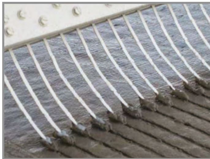
Longitudinal tining of a newly placed concrete surface
