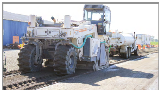
FDR with cement on a test track at UC Davis
