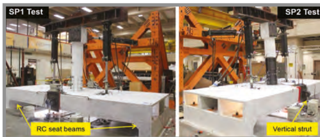
Cap beam, box-girder, column subassembly before bidirectional cyclic tests (left). Identical column repaired using a rapid carbon-fiber-reinforced polymer method during testing (right).
