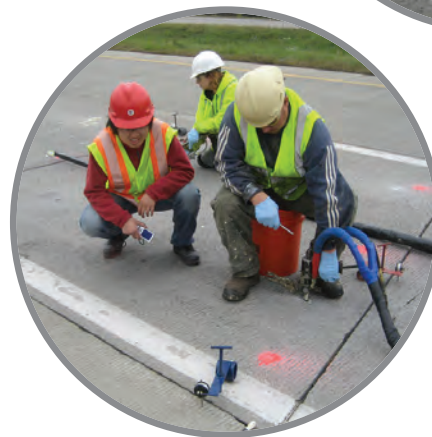
Field testing an injected, high-density polyurethane foam-stabilized base under concrete pavements
