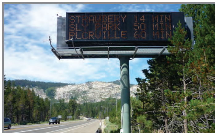
The travel time information is transmitted to changeable message signs and the Quick Map website.
