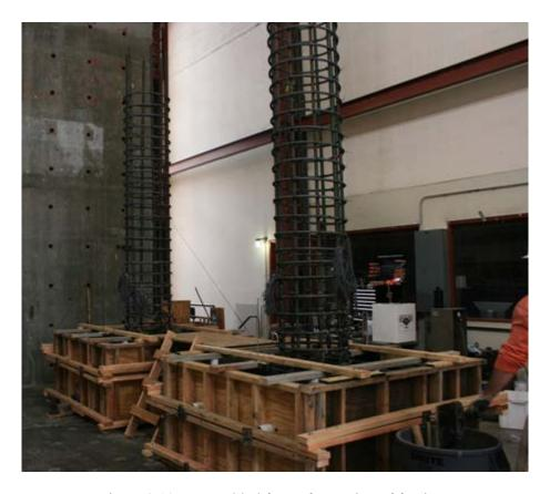
Figure 2.19 - Assembled forms for casting of footings
