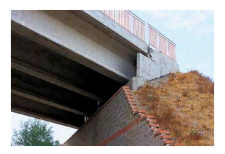
Figure 2.3. MSE bridge abutment at Estribo Francisco Mostazal site after 2010 Maule earthquake (Yen et al. 2011).
