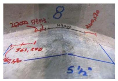
Figure 7.14: Fatigue Crack at Bend 8
