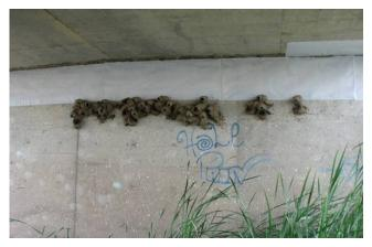
Figure 16. Completed nests below the bottom edge of PTFE treatments on a pier wall.
