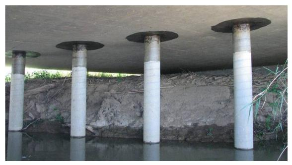
Figure 4. Highway structures with paint surface modification.
