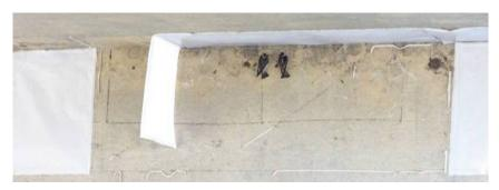
Figure 15. PTFE sheets detaching from the highway structure surfaces and cliff swallows building nests.
