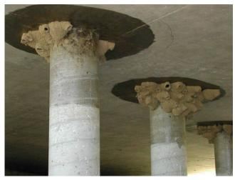
Figure 8. Completed nests on columns and overhead surfaces treated with silicone paint.
