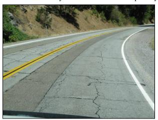
Figure 2.1: Alligator B and C cracking and digouts.
