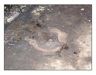
Figure 4.31: 605FD: Fines pumped from holes drilled for presoaking.
