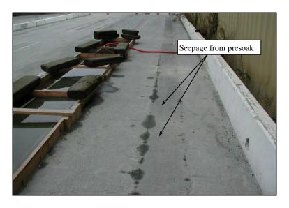
Figure 4.3: Seepage during presoaking.
