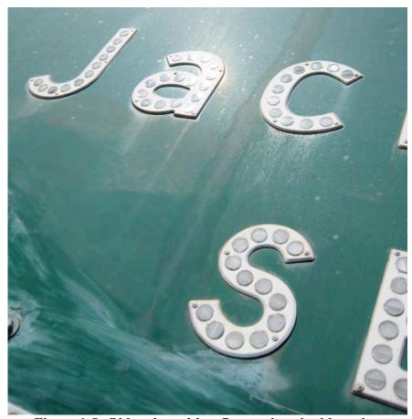
Figure 1-8: Older sign with reflectors in raised lettering
