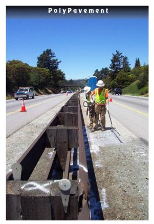
Figure 2.1 Caltrans workers applying PolyPavement weed barrier
