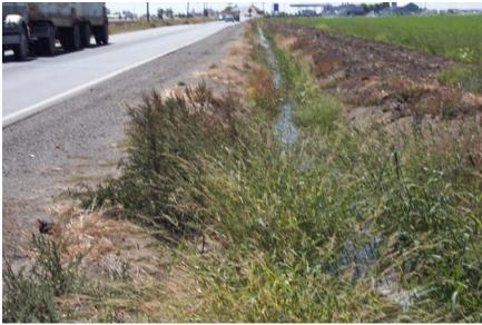
Figure 1.5 V-type Ditch With Irrigation Water
