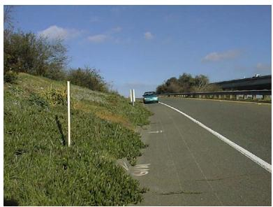
Figure 1.3 Ice Plant Growing Onto Right-of-Way
