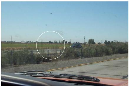
Figure 1.4 Undesirable Vegetation Around and Under Guardrail
