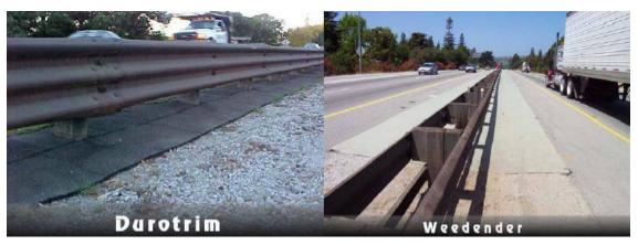
Figure 2.2 Different weed mat products tested on California highways
