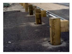
Figure 2.11 Asphalt concrete hardscape
