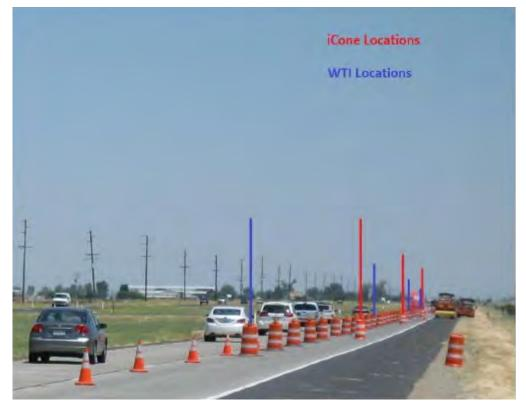
**Figure 15:** Typical May 14 – 18 iCone and sDrum Locations Note only six out of the normal 28 sDrums were deployed on 6/13/12 and 6/20/12.
