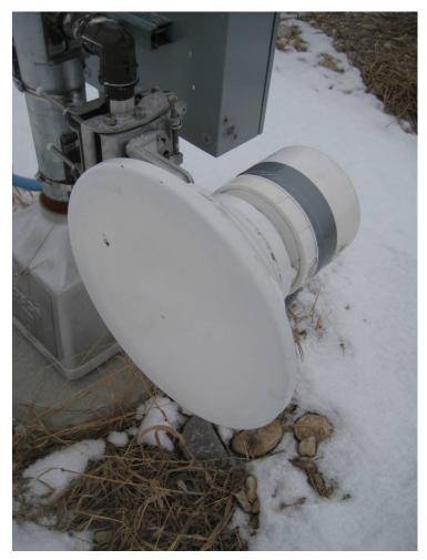
Figure 4.5. The receiver of the third generation break-the-beam system manufactured by ICx Radar Systems. Note: the transmitter looks similar to the receiver.
