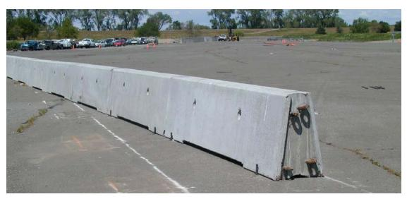
Figure 2-4 – Backside of Completed Barrier with Stakes
