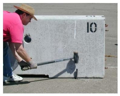
Figure 2-2 – Stake Installation
