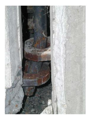
Figure 2-16 – Close-up of Bent Pin at Joint 8-9
