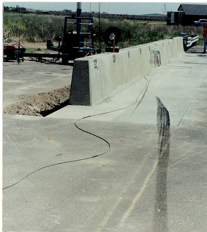
Figure 2.12 - Test 511 Downstream View Of The Type 70 Barrier
