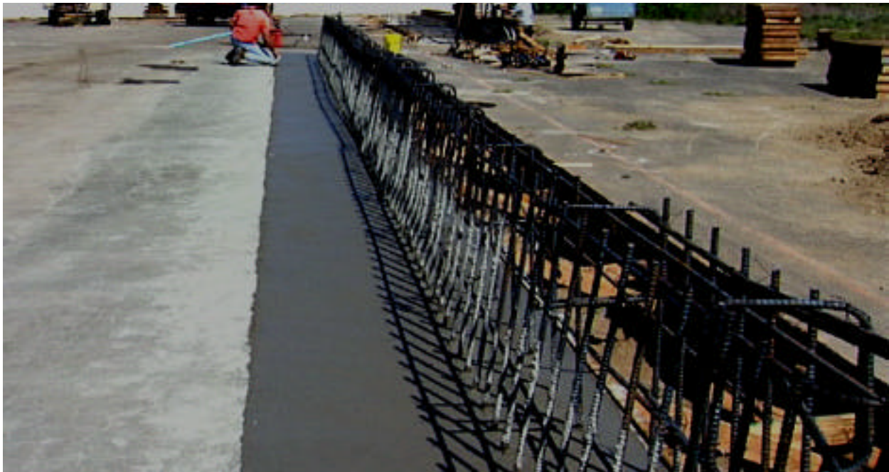
Figure 2.2 - Reinforcing Steel (From The Front)
