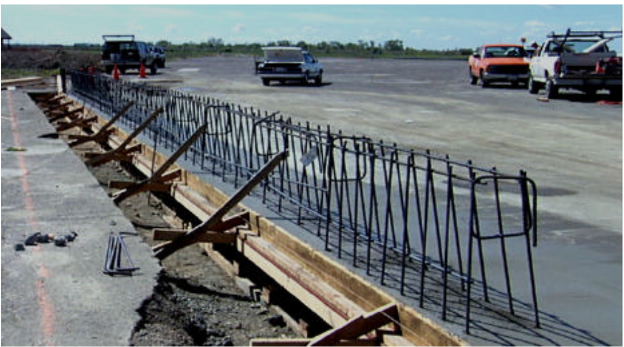
Figure 2.3 - Reinforcing Steel (From Behind Barrier)
