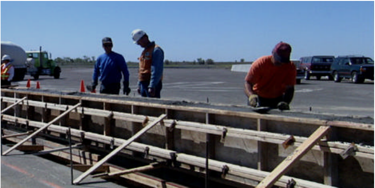
Figure 2.4 - Wood Forming And Finish Work
