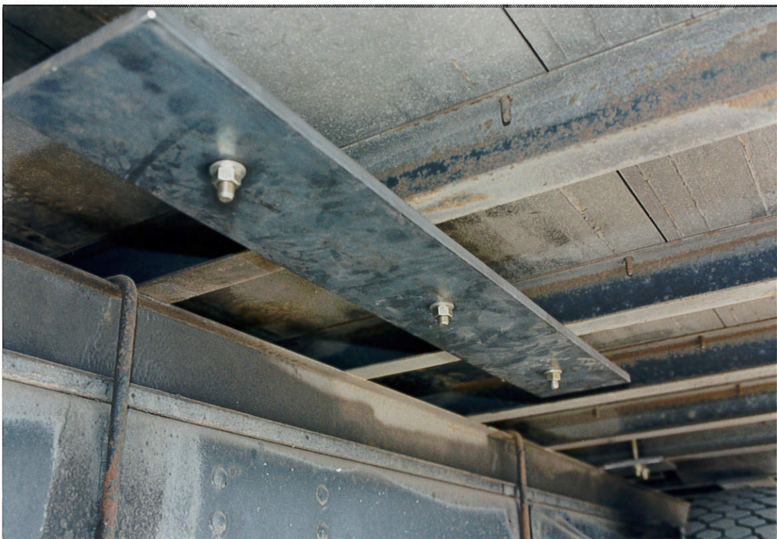
Figure 2.28 - Keeper Plates Used With The 150 mm Angle Iron on Test 513
