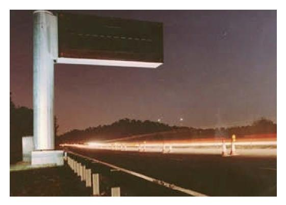
Figure 4 Composite Variable Message Sign Structure with Steel Post on the M25 Motorway in UK
