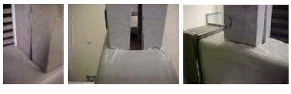
(b) (c) Figure 45 Cracking at rounded window
