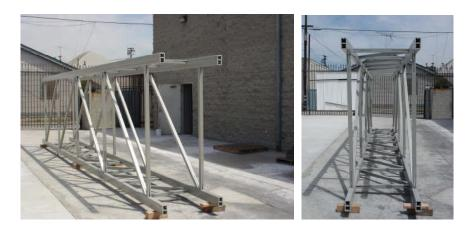
Figure 30 Trial assembly of Snap-fit Truss Structure for this Project
