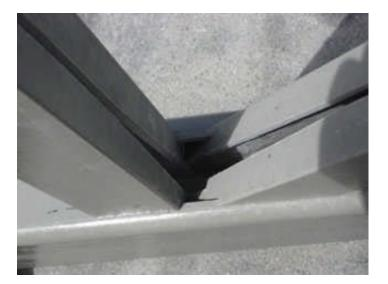
Figure 27 Detail Joint of Assembled Overhead Sign Structure The connection of the truss to the vertical pole is shown in Figure 28
