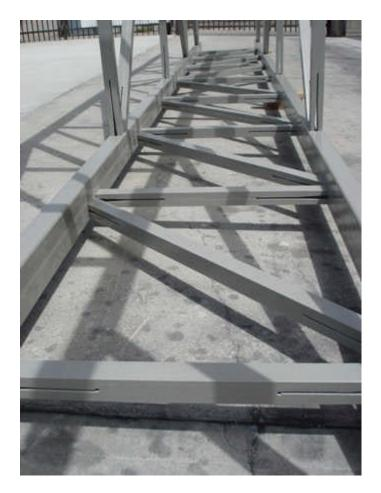
Figure 26 Assembled Overhead Sign Structure
