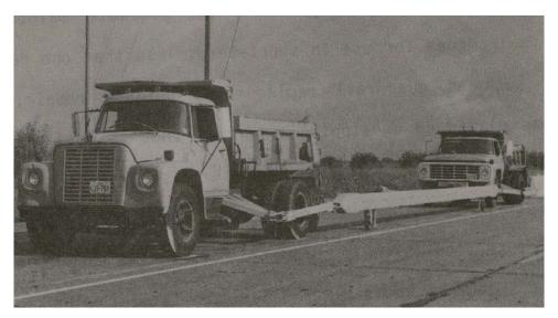
Figure 1-2 Truck-Mounted Portable Barrier
