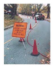
Figure 2. Typical Perimeter System Using Pneumatic Tubes<sup>[3]</sup>
