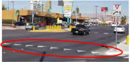
Figure 30. Example of "Advanced Yield Warning" (Source: http://safety.fhwa.dot.gov/ped\_bike/tools\_solve/ped\_scdproj/webinar052809/las\_vegas/)
