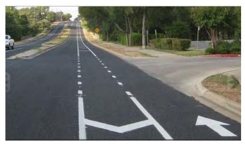
Figure 19. Example of "Buffered Bike Lanes"
