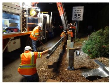
Figure 26. A Rail Truck Being Used to Install Rails onto New Posts.
