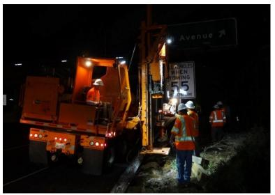
Figure 25. View of the Pounder Truck as it is Auguring a Hole to Place a Post.
