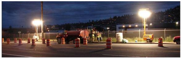
Figure 3. Balloon Lighting at a Highway Work Zone.
