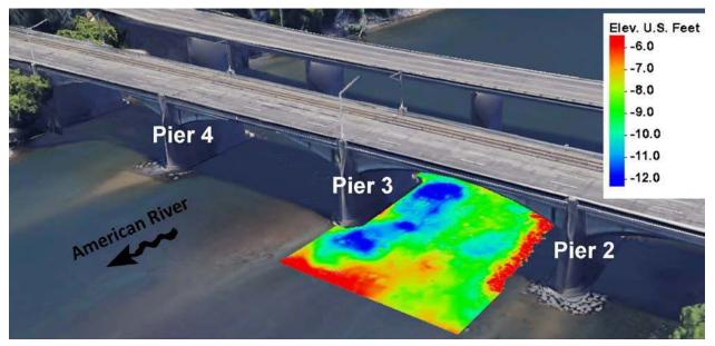
Figure 3.25: Underwater excavation before RSP installation at American River SR160 westbound
