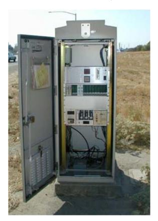
Figure 2-1. Type 334C Controller Cabinet Configured for CMS Operation
