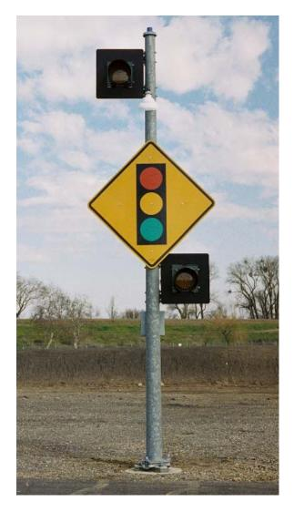
Figure 2-5. Warning Sign with Flashing Beacons
