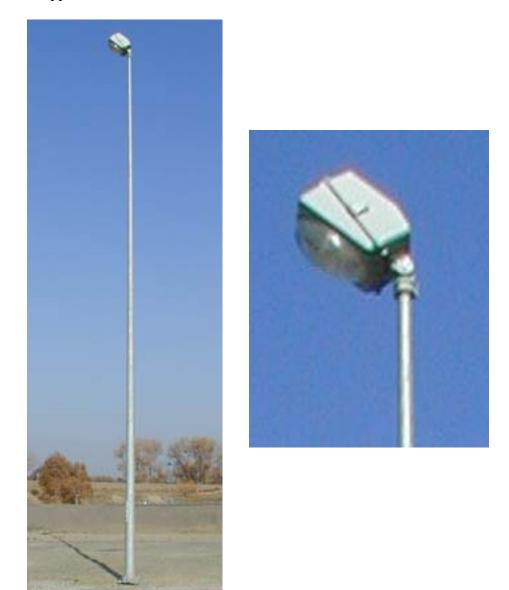
Figure 2-6. Pole Top-Mounted Luminaire (Overall View and Close-Up View of Head).
