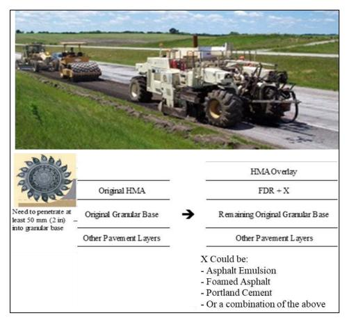
Figure 7. FDR construction process (Van Dam et al., 2015)
