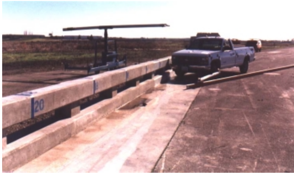
Figure 2-23 Vehicle and Bridge Rail before Test 545
