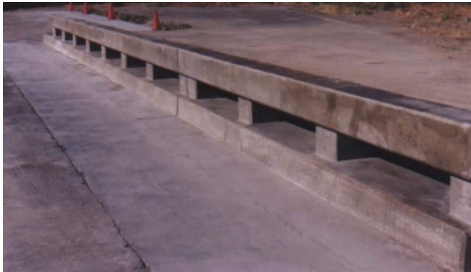
Figure 2-11 Completed Type 80 Bridge Rail
