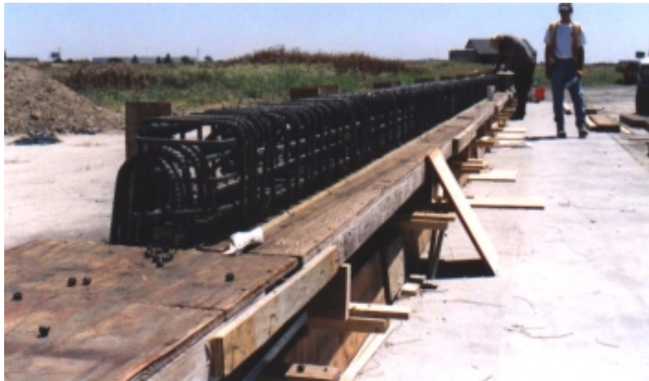
Figure 2-5 Steel Placement for Beam Section
