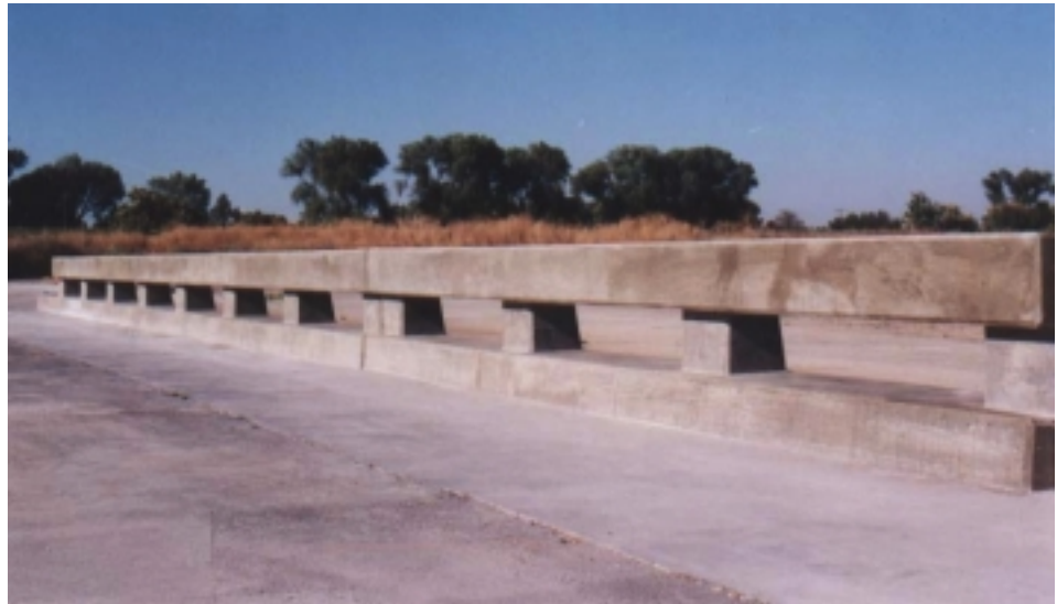
Figure 2-10 Completed Type 80 Bridge Rail
