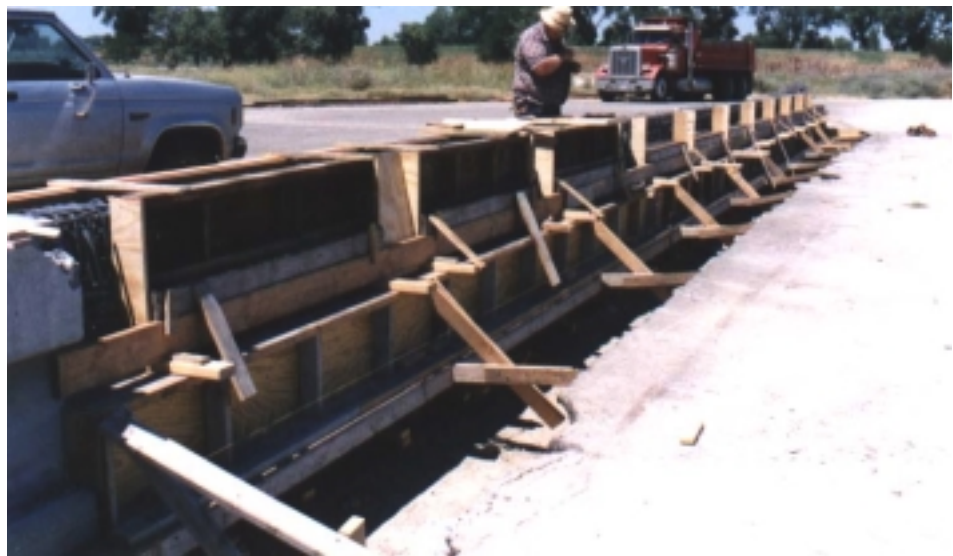
Figure 2-6 Form Placement for Beam Section
