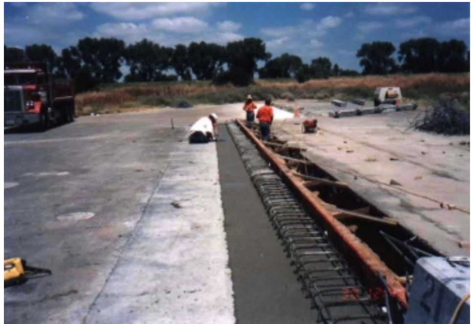
Figure 2-3 Simulated Bridge Deck Construction
