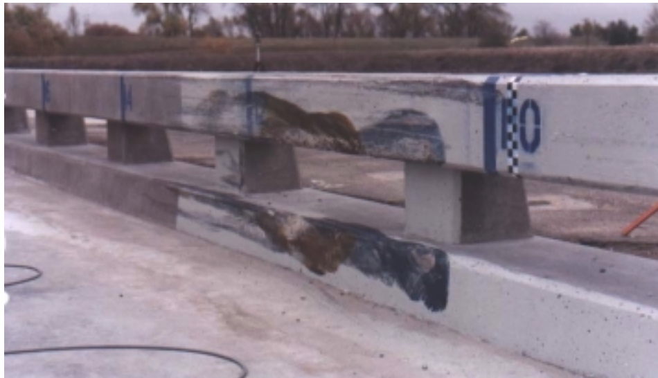
Figure 2-30 Test 545 Impact Area
