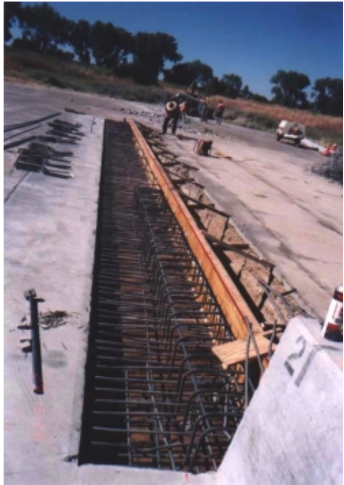
Figure 2-2 Concrete Anchor Block with Simulated Bridge Deck Reinforcing Steel
