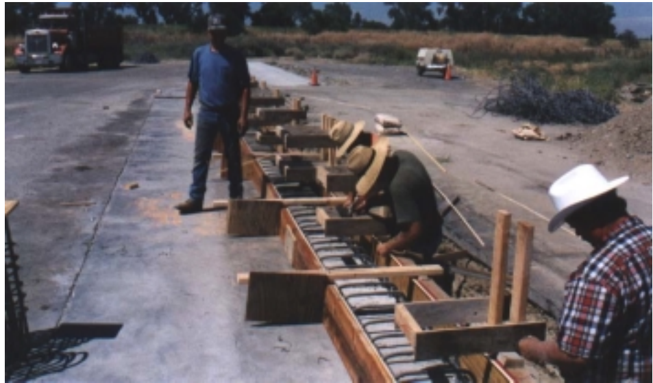
Figure 2-4 Form Construction for Curb
