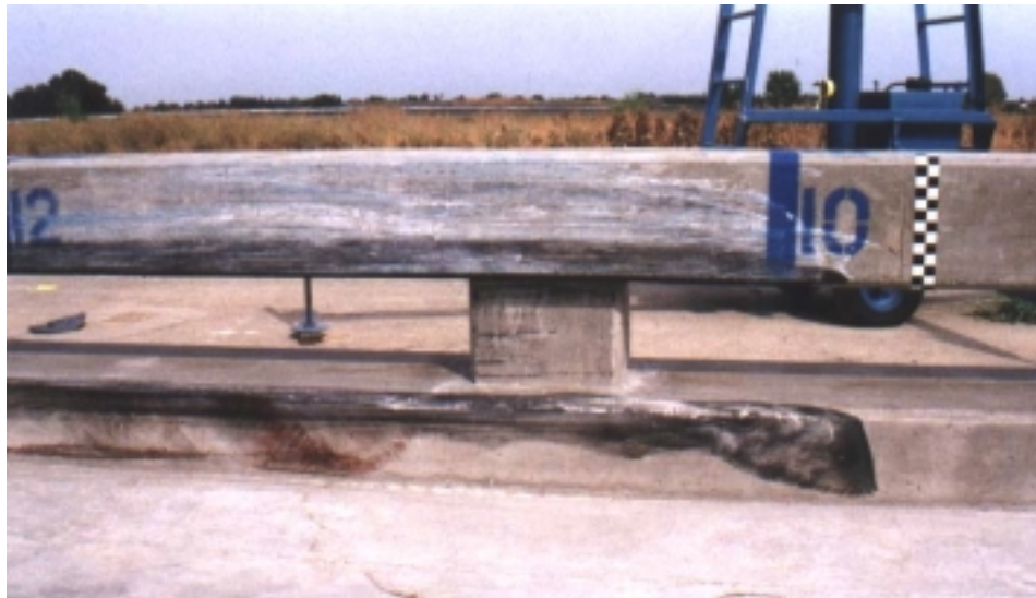
Figure 2-20 Post Impact Bridge Rail Scuff Marks Test 544
