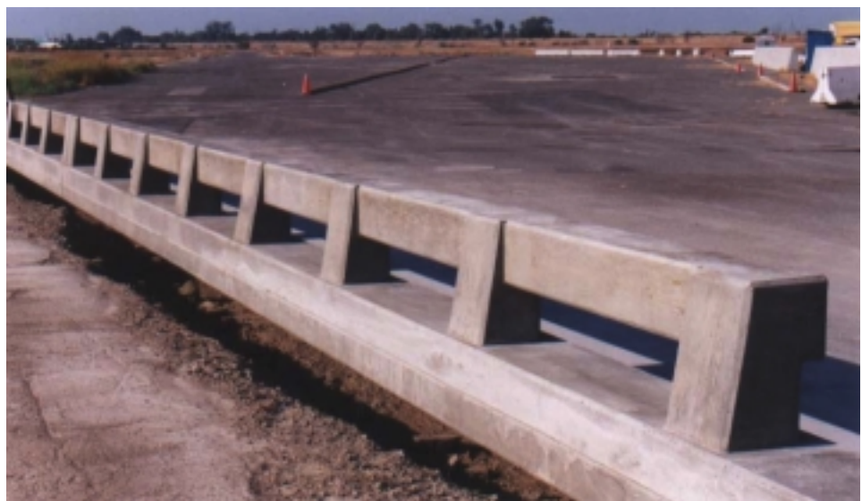
Figure 2-12 Backside of Completed Bridge Rail
