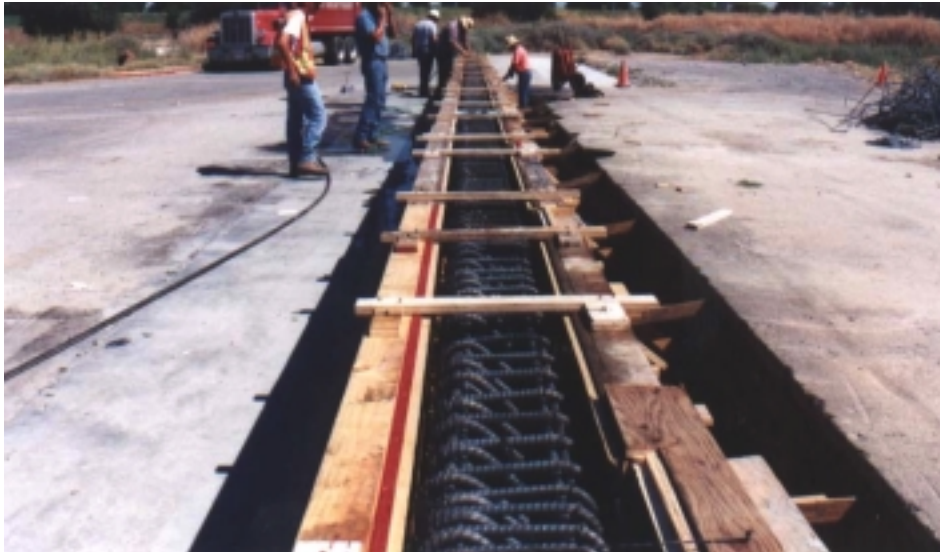
Figure 2-8 Top View of Forms for Beam Section
