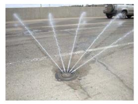
Figure 6. Bridge Deck Integrated Brine Spray
