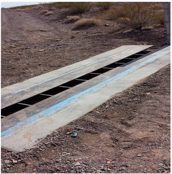
Figure 2. Permanent one-slot tortoise guard installed on a dirt road in Nevada. Note the escape route and connection to tortoise proof fence on the far side of the guard. Source: Clark County, NV.
