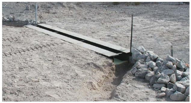
Figure 4. Installed temporary one-slot tortoise guard and fence. Note the escape ramps. Source: USGS
