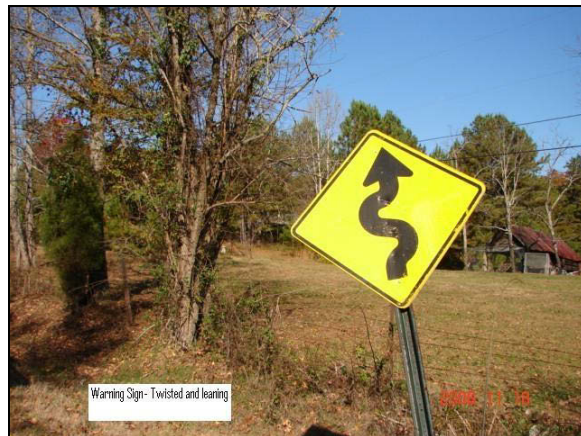
Deficient “Warning Sign” Sample – Count as Deficient
