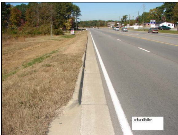
Functional Curb and Gutter Condition - Do Not Count as Deficient
