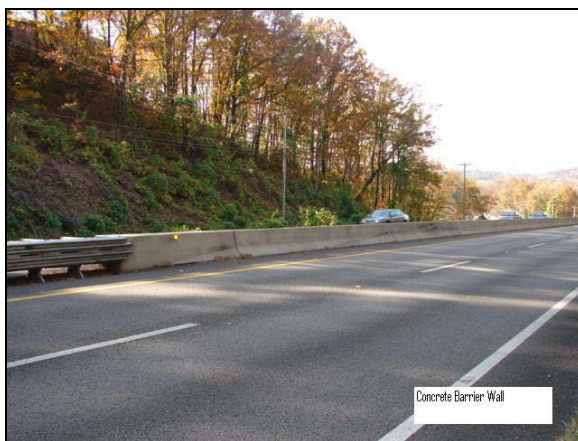
Functional Barrier Wall Sample – Do Not Count as Deficient
