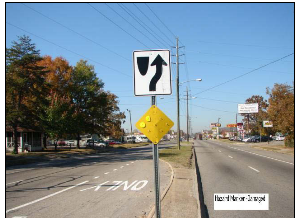
Deficient Object Marker - Count as Deficient
