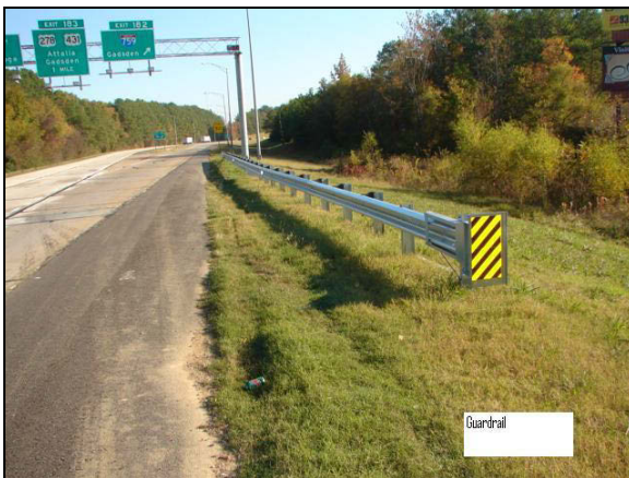
Functional Guardrail Sample – Do Not Count as Deficient
