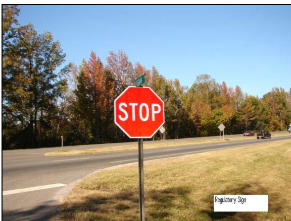
Functional “Regulatory Sign” Sample – Do Not Count as Deficient
