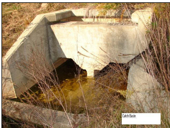
Functional Catch Basin Condition - Do Not Count as Deficient
