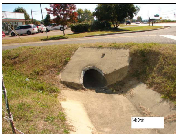
Functional Side Drain Condition - Do Not Count as Deficient
