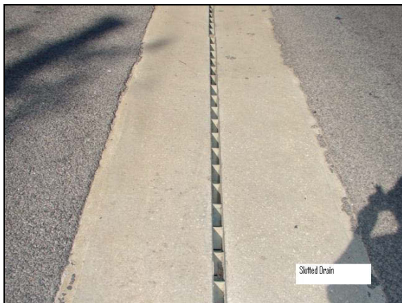
Functional Slotted Drain Condition - Do Not Count as Deficient
