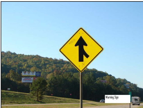
Functional “Warning Sign” Sample – Do Not Count as Deficient
