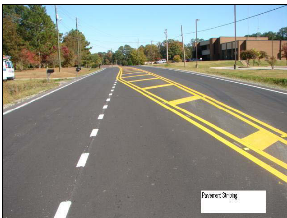
Functional Pavement Striping Sample – Do Not Count as Deficient
