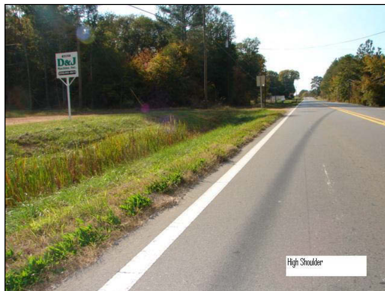
Sample Unpaved Shoulder, High Shoulder
