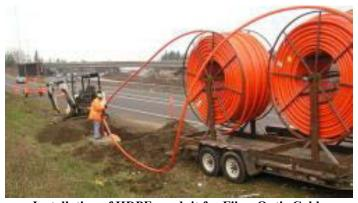
Installation of HDPE conduit for Fiber Optic Cable
