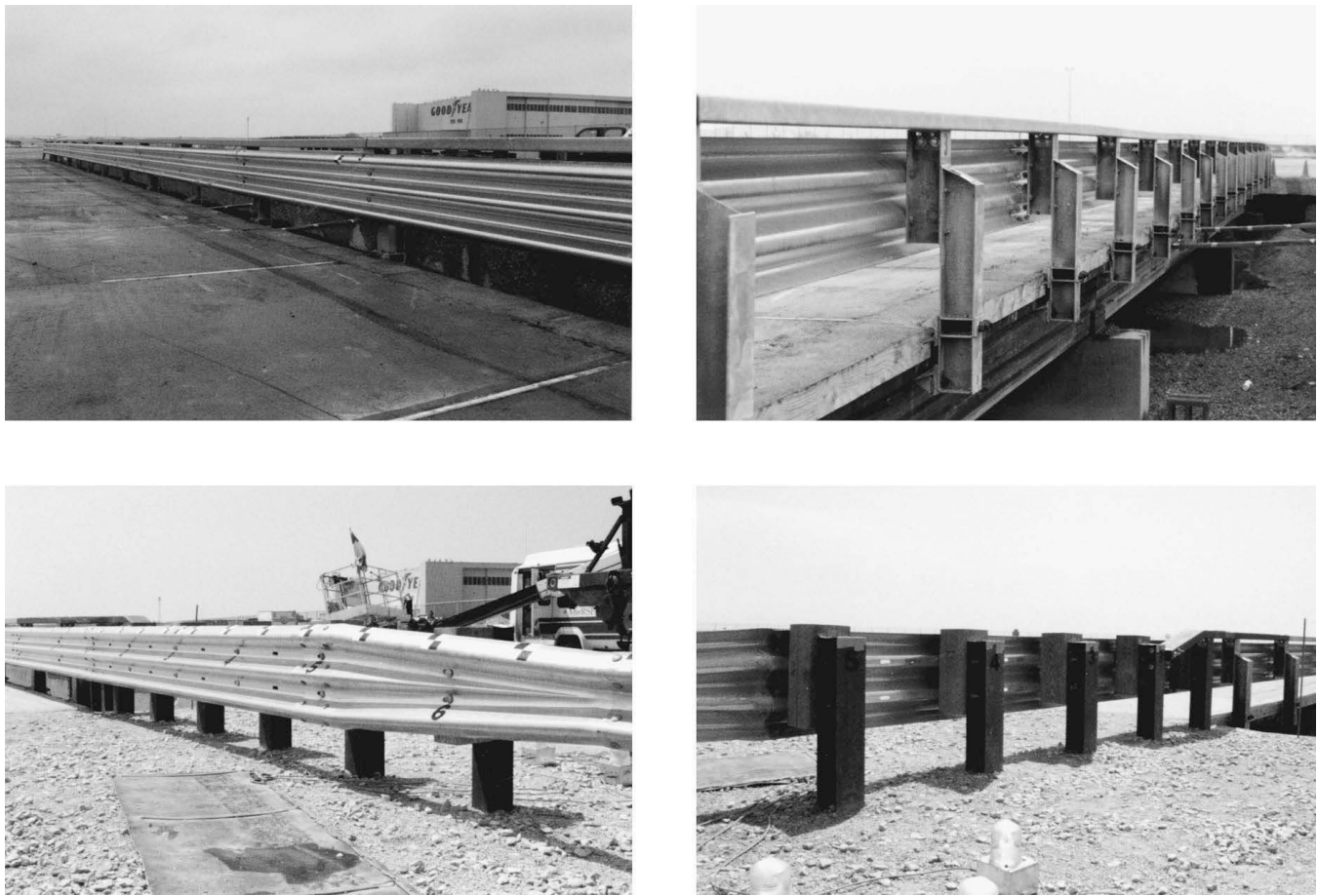
FIGURE 2 System No. 2: steel thrie beam with tube bridge railing ( top ) and thrie beam with tube transition ( bottom ).
