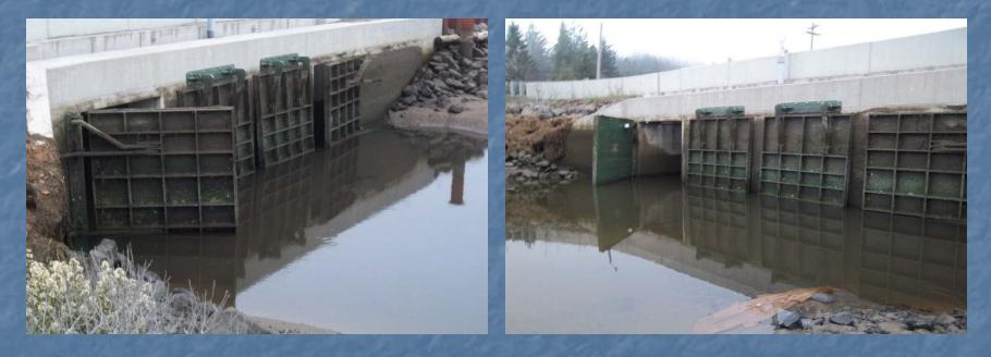
Top Hinge Side Hinge Array with MTR
