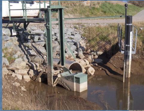
Small note: Failed culverts and SRT have been replaced with sidehinge gate and MTR, mark on bank at target inundation level Tidegate & MTR system at slack low-Tide.
