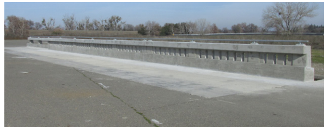
Image 2: Type 86H Concrete Barrier looking North East
