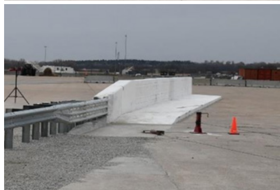
Image 1: Approach Guardrail Transition with Sidewalk
