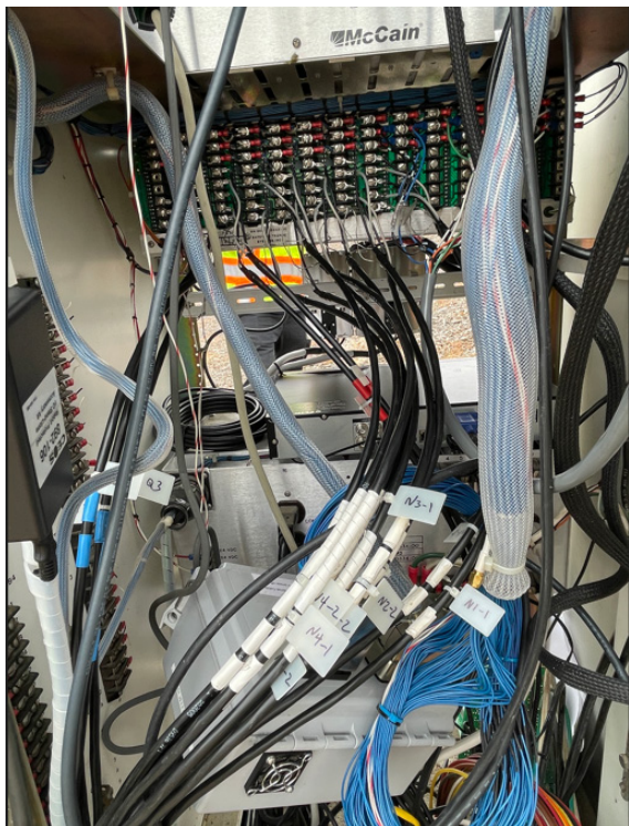
Image 3: The C1 Reader (grey box in lower foreground) installed in the North Main Street count station cabinet
