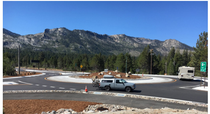
Image 1: Pictured is a roundabout located at the intersection of State Route 89 and US 50 in Meyers, California. Meyers is home of the Washoe Tribe and this roundabout was installed to slow driving speeds and reduce pedestrian incidents.
