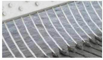
IMAGE 3: Longitudinal tining of a newly placed concrete surface
