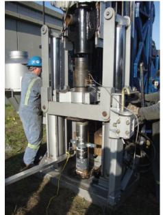
IMAGE 1: Drill ring with driving hammer in upward position
