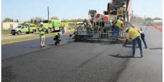
Figure 1: Rubberized warm mix asphalt paving at the Pavement Research Center
