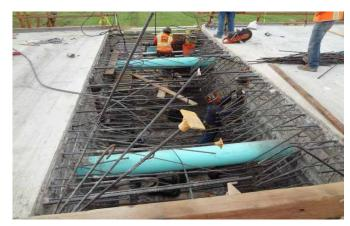
Image 2: Construction of an in-span hinge (Del Paso Park Overhead, Sacramento)
