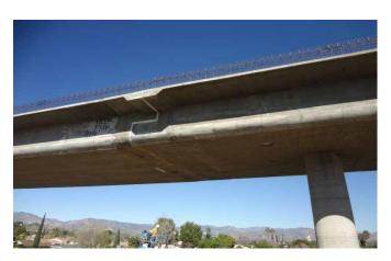
Image 3: In-span hinge of CIP/PS box girder bridge (N170-N5 Connector, Los Angeles)
