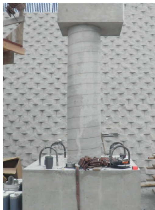
Figure 2: Completed cast-in-place column model
