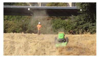
Figure 3: RCM mowing downward from top of 2:1 slope
