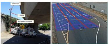
WWD VIPS installed at SB SR-51 & T St detection zones at WB US-50 & S River Rd
