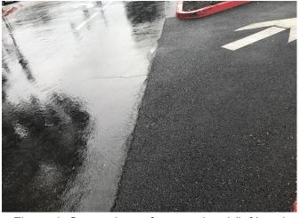
Figure 4: Comparison of conventional (left) and fully permeable asphalt pavement (right).
