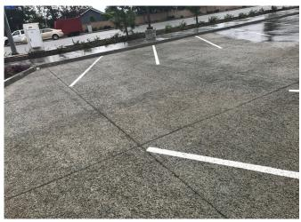
Figure 5: Fully permeable concrete pavement
