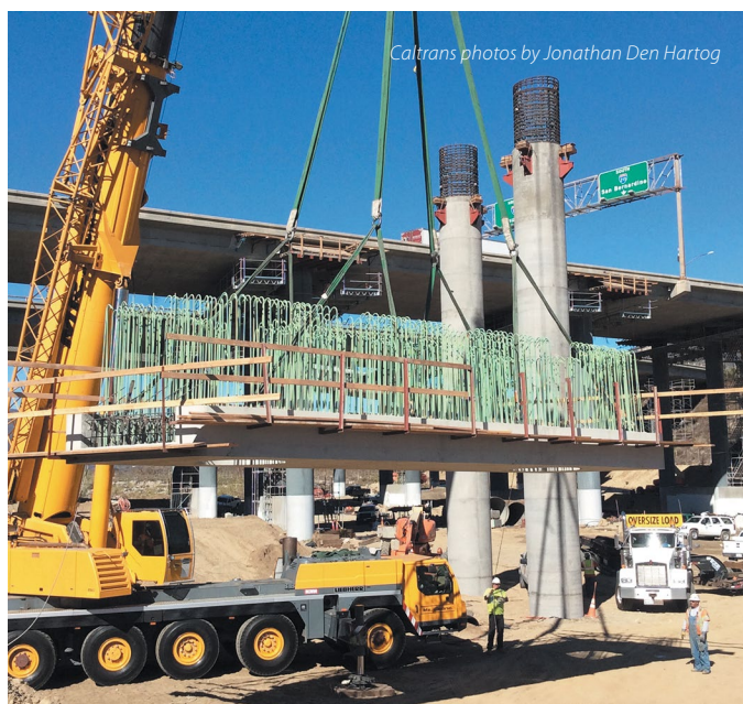
The Devore Road overcrossing bridge deck is lifted into place prior to the concrete pour as part of the interchange construction.
