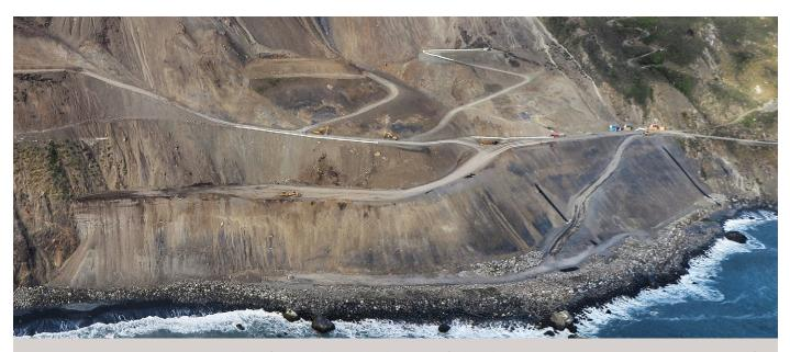
Construction crews create a new roadway base for the middle and north sections of the Mud Creek project. Access roads have been constructed for future maintenance of the site. A rock barricade, called a revetment, was built along the shoreline to keep the tide from eroding the embankments.
