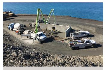
Crews pour a concrete drainage pad under the five-foot-plus diameter pipe that will drain excess water from the Mud Creek area.
