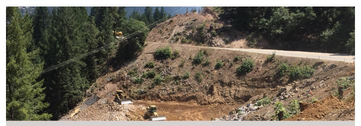
Construction crews fortified this embankment along SR 36 on the east end of the project. The contractor used rock from the work site for slope protection and drainage basins, eliminating the need to haul in material from other places, saving time, money and reducing air pollution.
