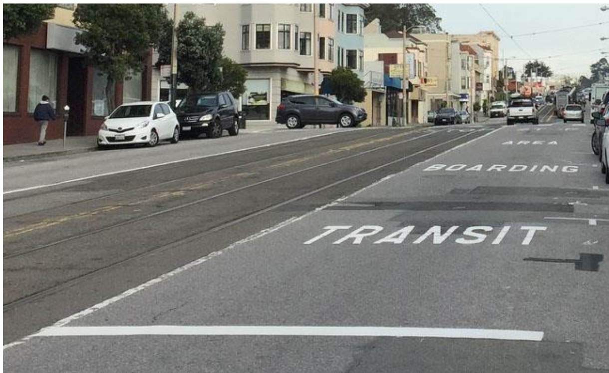
Figure 4. New Pavement Markings
