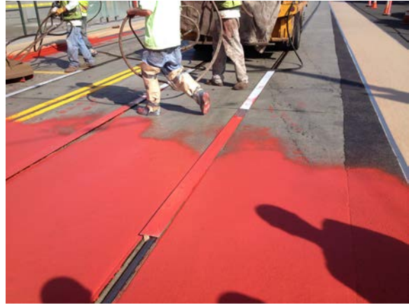
Application of Spray Coating
