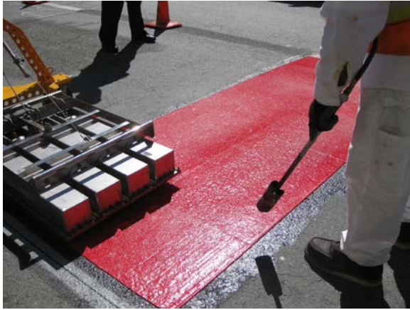
Application of Preformed Thermoplastic
